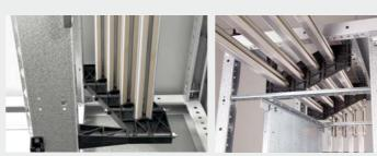
**Sloping Smart-Energy:** busbar system placed on the cable housing W= 300 and W=400 and on the top.
