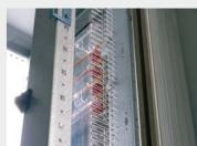
Vertical dividing panel: possibility of dividing the cabinet between circuit breakers space and cable housing.
