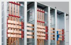
**Cabinet – rear busbars:** cabinet with sections and segregation form 3b. Vertical and horizontal busbar system placed at the back.
