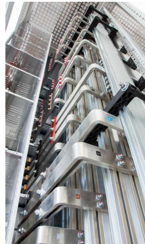
Circuit breaker connection to vertical busbars
